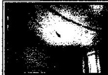
Plastic covering leaking ceiling in tenant's bedroom . Dark spots are mould, the bulge is water accumulated in the plastic.
